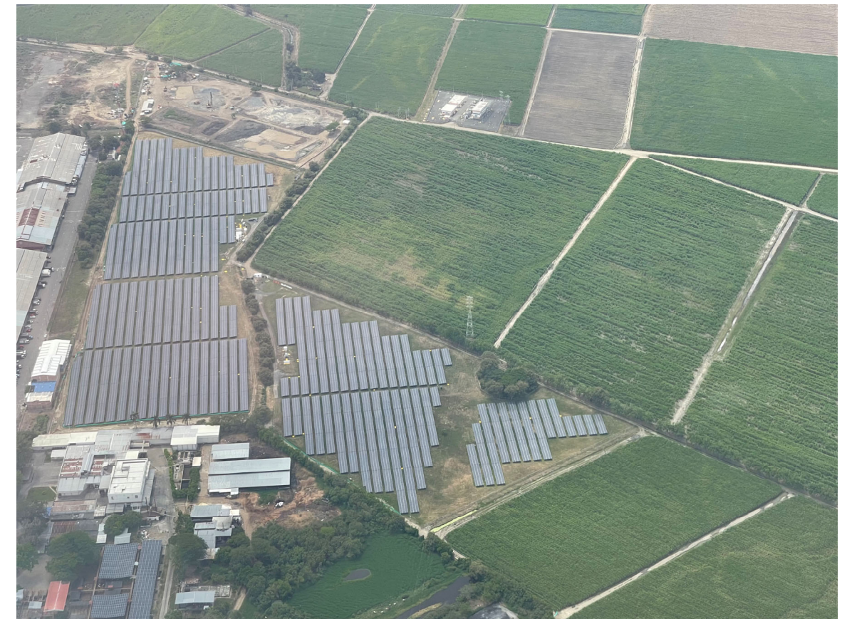
Solar Power near airport, Cali, Colombia
