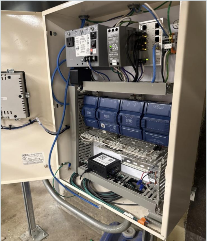
Field installation: Super SkyBox in installed in controls panel
