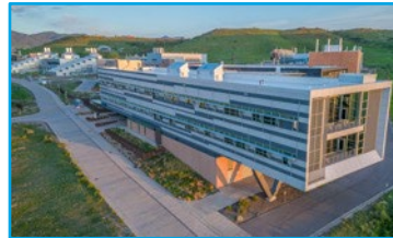
Energy Systems Integration Facility
